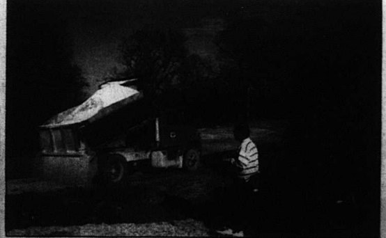
The Rockcastle County road department gravelled a portion of the Toddy Payne Road at Pine Hill Wednesday morning. In the photo is landowner Mike Gates who wants the road closed.
