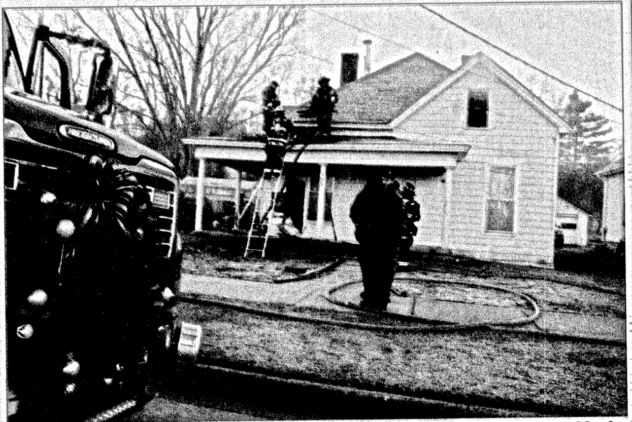
The Mount Vernon Fire Department responded to this house fire on West Main Street Monday morning but the fire was detected before the home was destroyed, officials say. Damage inside was extensive in some areas. The cause of the blaze is unknown at this time. No injuries were reported. The wreath on the fire truck demonstrates the need for first responders to remain on duty during holiday seasons.
