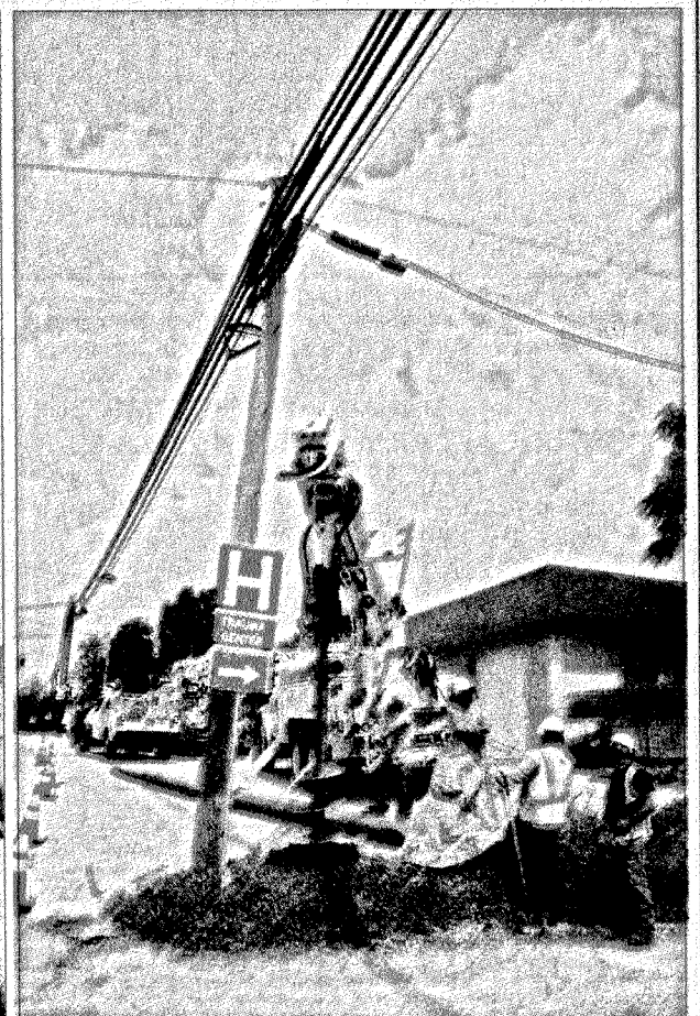
Workers with Kentucky Utilities set a new pole on Highway 150 near Main Street Monday after a construction worker broke the existing pole with the boom of a back hoe. Electric was out on both sides of West Main Street for nearly seven hours causing businesses to close for most of the day. Shown at left is the broken pole and at right, workers drill the hole for the new pole.
