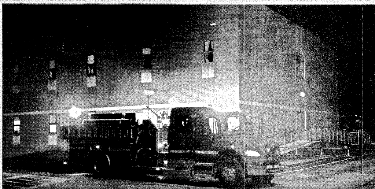
The Mount Vernon Fire Department was called to the Mount Vernon Elementary School Friday night after smoke was reported in the building. Once on the scene, first responders learned the smoke was from a faulty heating and cooling system and no fire had occurred. Fire fighters ventilated the building and no damage was reported from the smoke.
