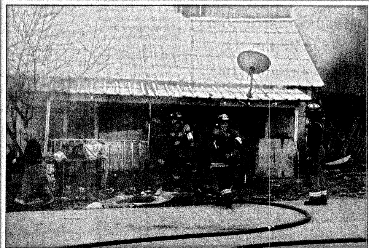
First responders rescued a dog from an abandoned home on McHargue Branch Road after a fire broke out Wednesday morning. Officials do not know the cause of the fire but neighbors say that sometimes homeless people stay in the house. Volunteers of the Mount Vernon Fire Department kept the flames from spreading to the house next door. No injuries were reported.
