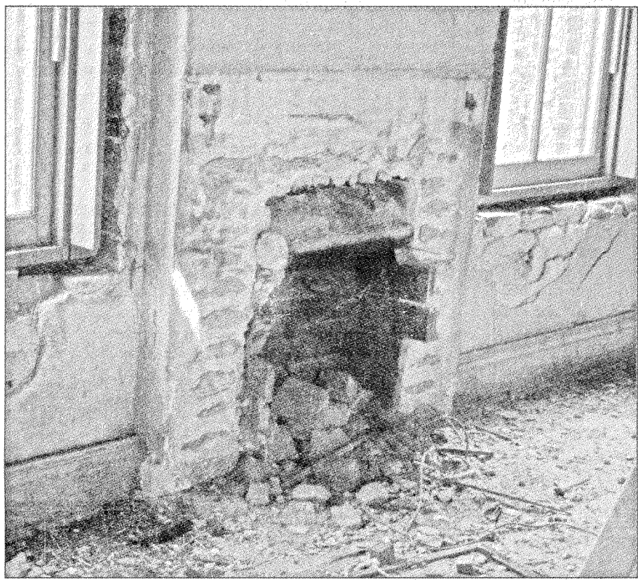
Some of the brickwork is badly delapidated inside the Jones Building but workers are hoping to keep as much of the original structure as possible.
