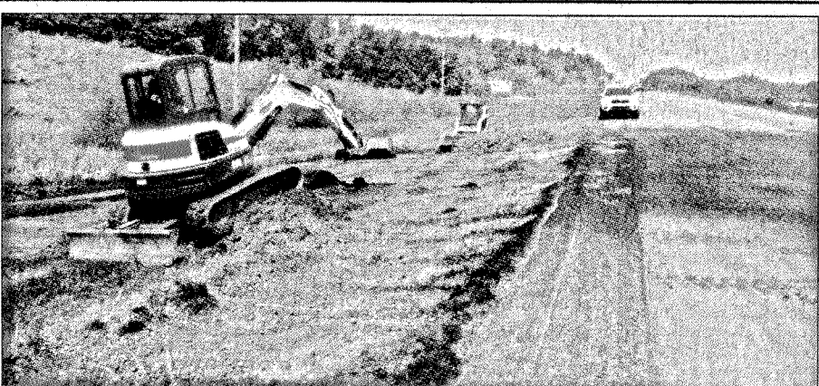
Workers from the Kentucky Transportation Cabinet spent over 24 hours cleaning and repairing the damage caused by a two vehicle accident Sunday on Highway 150 after a fuel truck, which had collided with a car, overturned, spilled fuel, burst into flames and melted blacktop. Crews opened the roadway after about 10 hours but are still working to clean up the fuel that spilled into the ground around the accident.
