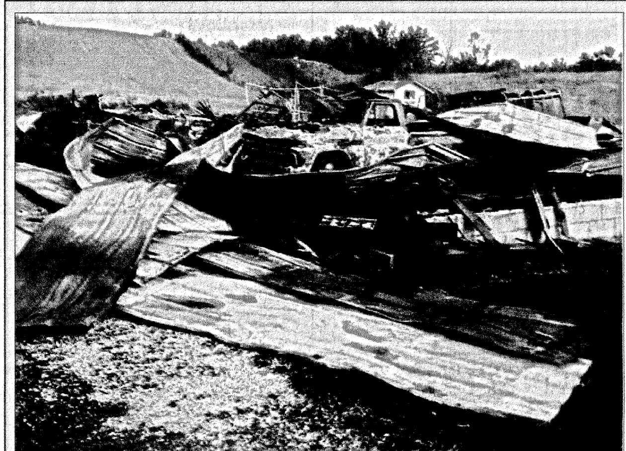
A barn owned by Gary and Vickie Scott near the Rockcastle/Lincoln County line was completely destroyed by fire Monday morning. Officials say the barn was fully engulfed in flames when they arrived at the scene. Investigators are looking into the cause of the blaze.
