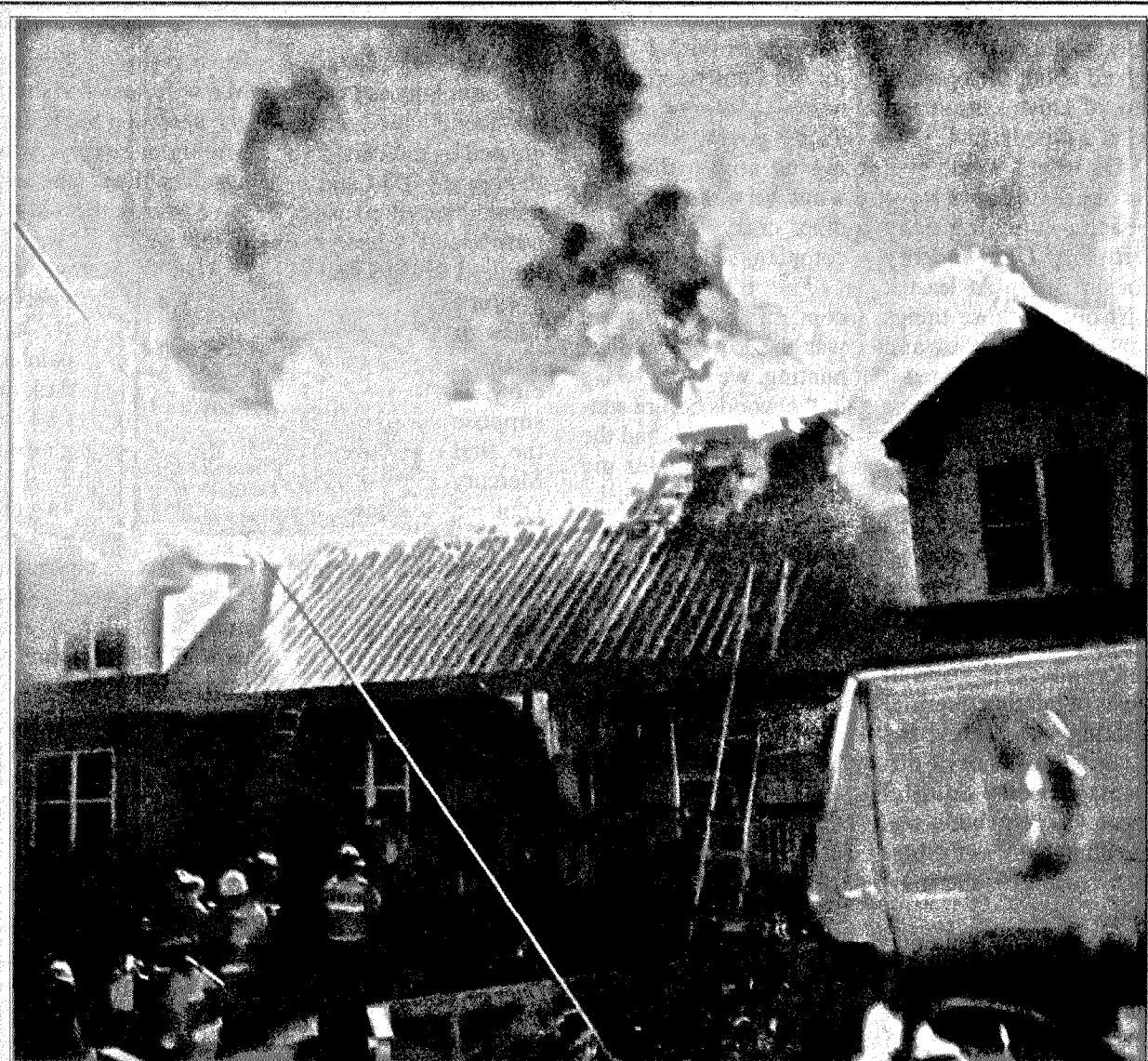
The home of Phil and Charli Fox on Otter Lane in northern Rockcastle County suffered heavy damage after a blaze started near the attic space in the early hours of Monday morning. Officials with the Brindle Ridge Fire Department originally thought someone might be trapped inside. Firefighters made rapid entry into the structure but reports say no one was inside. Officials say all firefighters from different departments in the county worked well together to save the structure. Those on the scene were the Brindle Ridge, Mount Vernon, Brodhead, Livingston and Berea Fire Departments, Rockcastle EMS, Rockcastle Sheriff's Department, and the Kentucky State Police Fire Investigators. Though one firefighter was injured at the scene, his injury was not due to the fire. The cause is not known at presstime.
