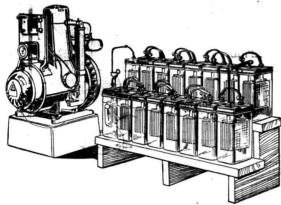
It consists of an engine, generator and switchboard built as a compact unit. This unit with the storage battery comprises the complete equipment.
