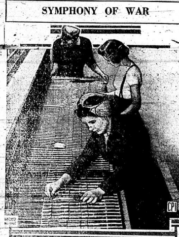
—Passed by Censor— It looks like a xylophone but it's a row of Bren gun barrels being reloaded in a Toronto munition plant. Canada which made the weapons of this kind before the war now possesses a factory that has the largest output of any automatic gun plant in the world. Many of the workers in the plant are women and they have proved themselves to be adept in this kind of employment. All the requirements of the Canadian armed forces are being met by this one factory and large numbers of Bren guns are being supplied to Great Britain. For these guns and many other munitions required by Great Britain, Canada is finding much of the money. During Canada's present fiscal year, the Dominion expects to finance British war purchases in Canada to the extent of $1,500,000,000, which is equal to $25,000,000 in terms of American population and income. The Canadian taxpayers are providing the cash.
