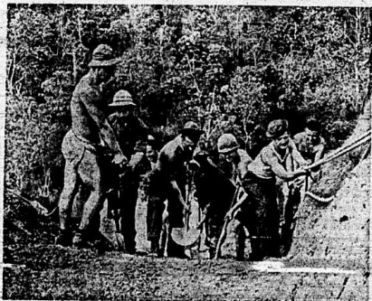
Building "Pee" roads in New Guinea is all part of the day's work for American army engineers. This particular road under construction near Port Moresby, main Allied base in New Guinea, is so steep that the men must hold on to ropes to keep from falling backward. The grade drops about 65 degrees behind them.
