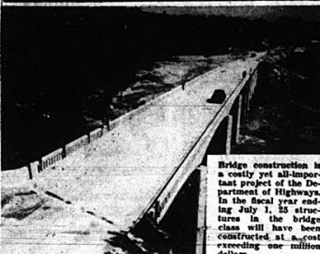
The bridge above is typical of the new spans being constructed by the department. The structure, named the James Todd Crawford Memorial Bridge, crosses the Green River on the S. 68 in Greenup County. It was completed at a cost of $307,000.00.
