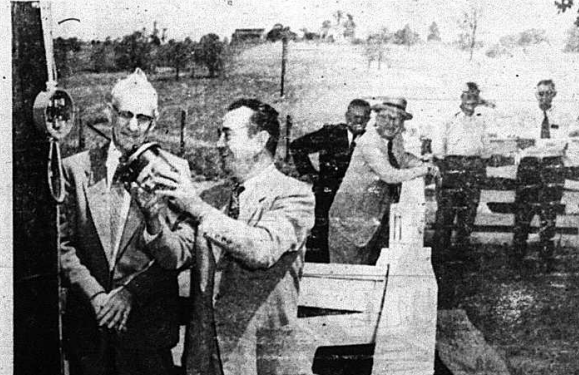
Governor Wetherby installing the electric meter during the celebration on the J. F. Rankin farm near Prescherville.
