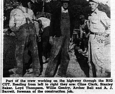
Part of the crew working on the highway through the BIG CUT. Reading from left to right they are: Gliese Clark, Stanley Baker, Lloyd Thompson, Willis Gentry, Archer Bell and A. J. Barret. Foreman of the construction job.
