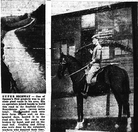
SUPER HIGHWAY — One of Spence's first projects was to get some good roads in his area. His co-operators joined hands to build this road in the Scaffold Cave-Roundstone area (seven miles total). They loaded rock onto their farms, wagon and designated days, hauled it to the road site; there the rock was broken by hand, and put on the road bed. Grading and filling also were done by the volunteer workers who donated their time, tools and material in most cases.
