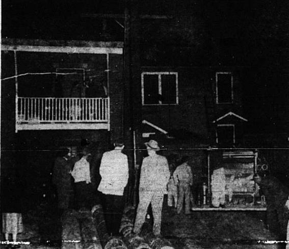
FIREMEN had to literally dig the fire out of the roof of the Post Office Building Sunday night. Firemen had to dig for nearly an hour before the fire, smoldering between the roof and ceiling of the second floor, was extinguished.
