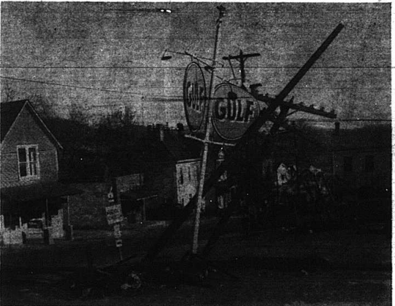
CORNER U. S. 25 AND U. S. 150 — A Truck Tangled With A Cable —
