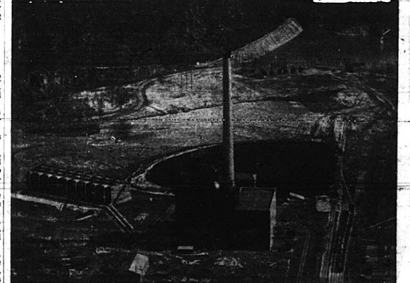
SOURCE OF ELECTRICITY—An aerial view of the Kentucky Utilities Co., E. W. Brown generating station at Dix Dam shows the plant with the coal pile behind it and the dam in the background. The cooling tower is at left and the spar track and substation at right. The first $25,000 kilowatt unit at the plant went into production this week. Mr. Vernon's electric supply will be furnished by the new plant.
