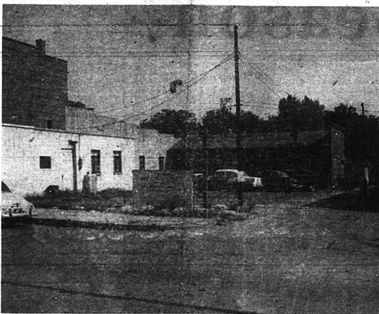
NEW POST OFFICE SITE—On this lot adjoining the former Bus Station Building and Bryant Bros., a new post office building is being constructed. Done by the work is Jack Crawford and associates. The building will face Main Street and will be stone and brick. J. H. Rowe is building the post office and will lease it to the Post Office Department.
