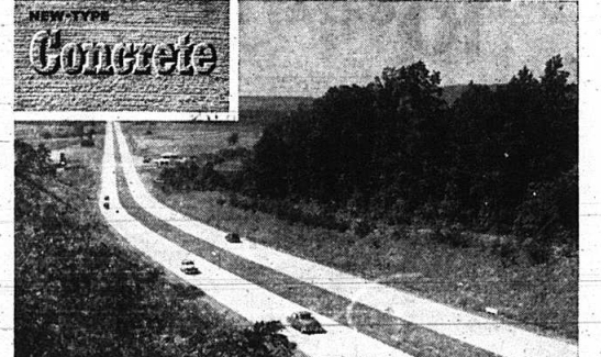
This new-type concrete road is smooth, quiet and comfortable
