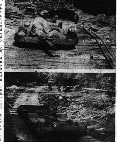
OUT OF A MOUNTAIN—These pictures were taken at the newly opened mechanical coal mine in the Skegg's Creek section in Southeast Rockcastle County. Top, one of the motors is shown just after pulling a load of coal out of the mine entrance in the upper right. Bottom, the motor and trailer return after a trip to the tippie in the background.
