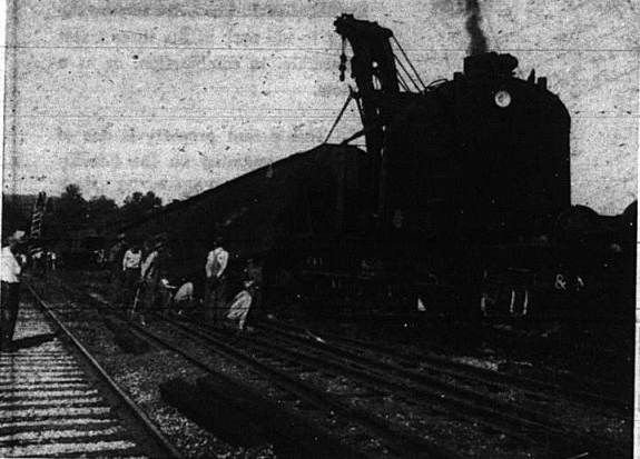
L & N ACCIDENT CAUSES $14,000 DAMAGE—An L & N Railroad accident near Wildie about 5 m. Sunday left 22 cars derailed and rolled up a total damage estimated at about $14,000. Some 50 men were still at work this week cleaning up the debris. A railroad official on the debris scene said the accident occurred when a north-bound train from Corbin burned out a journal on an axle—and left the track wrecking 17 cars loaded with coal. A south-bound train in the accident. The accident occurred about one-half mile south of Wildie. Two entire wrecks were called out to help clear the track of the wreckage.
