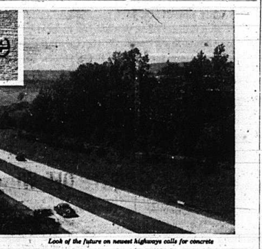
Look of the future on newest highways calls for concrete
