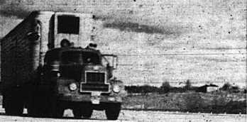
Modern concrete for Kentucky's Interstate 65 south of Elizabethtown
