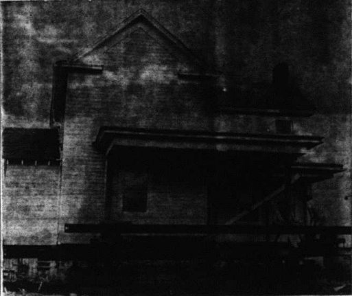
MOVING ALONG -- This house, owned by Gordon Graham, on Lovell Lane at Mt. Vernon, is being moved to an area facing Sevil Street. The house, previously owned by Ed Snee, is being moved by a Winchester firm. The house, in one piece, was moved about 800 feet, with no damage.
