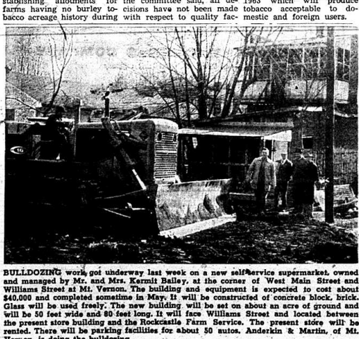
BUILDING work got underway last week on a new self-service supermarket, owned and managed by Mr. and Mrs. Kermit Bailey, at the corner of West Main Street and Williams Street at Mt. Vernon. The building and equipment is expected to cost about $40,000 and completed sometime in May. It will be constructed of concrete block, brick. Glass will be used freely. The new building will be set on about an acre of ground and will be 50 feet wide and 80 feet long. It will face Williams Street and located between the present store building and the Rockcastle Farm Service. The present store will be rented. There will be parking facilities for about 50 autos. Anderkin & Martin, of Mt. Vernon, is doing the building.
