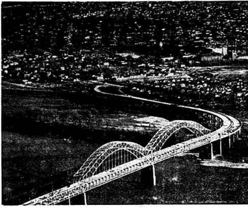
Kentucky's double deck Sherman Minton Bridge carrying Interstate Route 64 across the Ohio between Louisville and New Albany. It, won the American Institute of Steel Construction's award as the most beautiful long span bridge of 1962. Earlier winners of this high honor include the Golden Gate Bridge, the Mackinac Straits span and Rainbow Bridge over Niagara. On the Sherman Minton Bridge northbound traffic uses the upper level, southbound the lower.
