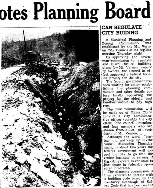
NEW WATER LINE - Mt. Vernon Water Works employees are shown digging a ditch to lay a 550-foot, six-inch water main along old US 25 to the residence of McKinley Arnold. Considerable blasting has been necessary to dig the trench.
