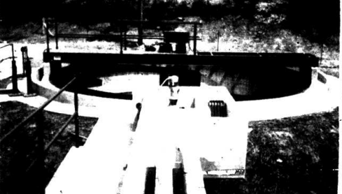
PRIMARY CLARIFIER - Into this bowl will go all sewage to be separated into solids and liquids and passed along to a disposer. In the foreground of the picture is a grider. An open house probably will be held at the plant after cut-over.
