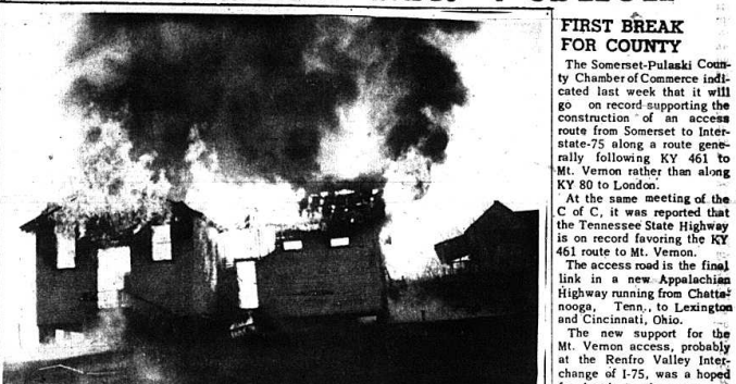
ORLANDO SCHOOL BURNS-- The Orlando School at Brush Creek was destroyed by fire about 7:30 a.m., last Thursday. The 55 children who attended the school are now attending temporary classes in the Flat Run Baptist Church until two mobile units arrive. Since most "one-room" schools are gradually being abandoned by the school system, it is doubtful the building will be reconstructed.
