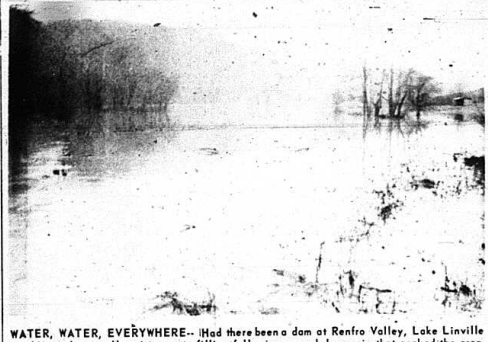
WATER, WATER, EVERYWHERE-- Had there been a dam at Renfro Valley, Lake Linville would have been well on its way to filling following a week long rain that soaked the area. The above picture was taken from the bridge over Renfro Creek.
