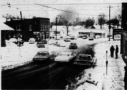
ONE LANE TRAFFIC-- Motorists had only one lane open in downtown Mt. Vernon early Saturday morning following one of the heaviest snowfalls of the year, plus the added rush of holiday traffic. The curbs on the left and right of Mt. Street were abandoned during the night when they became stalled in the snow.
