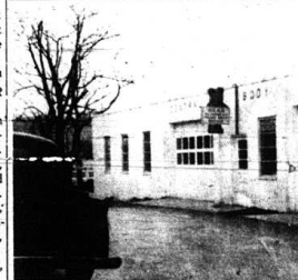
NEW BUILDING COMPLETED -- Johnny Eston, Mt. Vernon mechanic and auto body repairman, has constructed a new garage building adjoining Jerry's Practice House at Mt. Vernon. The concrete block building overlooks the L & N Railroad. Mr. Eston is now open for business.
