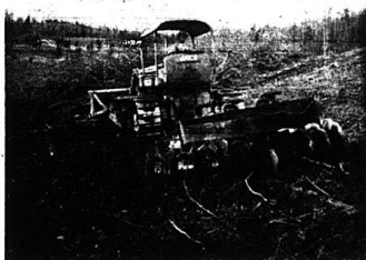
Another D-6 tractor with hydraulic angle blade is just the right size dozer for farm ponds, waterways, roads, and any other type of work that you need a dozer on.
