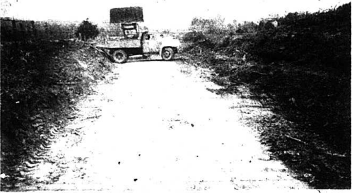
WIDENING OF ROAD -- The State Highway Department is in the process of widening about three miles of the Purr-Rigsby Road in the Brindle Ridge section of the county, according to John Houston, State Highway Supervisor for Rockcastle County. The road will be widened to 36 feet between the drain ditches and will in the future be paved with a 24 foot surface.
