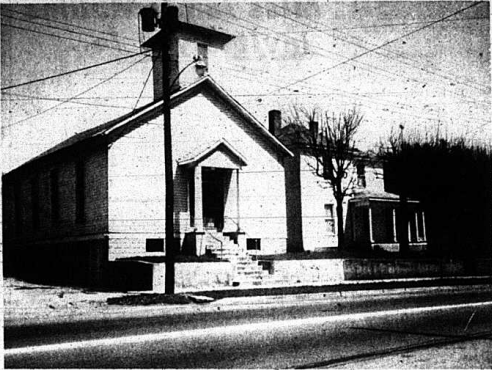
74 YEARS OLD- The Livingston Christian Church, shown in the above photo, has been torn down and a new church, on the old foundation, is in the process of being erected. The building was built in 1893 when the church was first organized. Bro. Robert Waddie is minister of the church. The house, located adjacent to the church, is the former residence of Mr. and Mrs. G. D. Cook. Mr. Cook was the first Sunday School Superintendent of the church.
