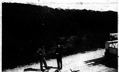
C. H. Webb of Livingston, right, and Floyd Gabbard, of Brodhead, Maintenance Supervisor for Jackson County R.E.C.C., stand on the Rockcastle River Road where the dual bridges of Interstate-75 will cross Rockcastle River in Laurel and Rockcastle Counties. These grade-and-drain bids will complete the ones to be let for Rockcastle County. R.E.C.C. workers are shown burying their electric cables under where I-75 will be constructed into Laurel County.
