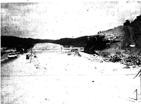
SPAN THE GAP. —The U.S. 25 overpass at Burr has been completed. Soon motorists will have new "old" U.S. 25 to travel on as the present U.S. 25 will be filled for a bed for the Interstate.
