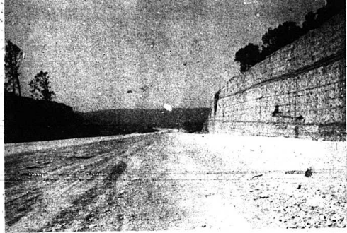
I-75 BY-PASS PROGRESSING: The above photo shows the I-75 By-Pass looking north from near Barr. Grade and drain on this section is nearing completion and paving will begin in the near future. The bottom photo is looking south from the Renfro Valley area. According to J. P. Noonan, District Highway Engineer, the By-Pass is scheduled to be opened November 15.
