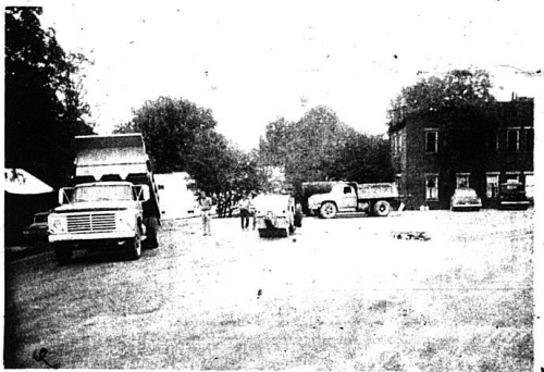
READY FOR USE-- The Mt. Vernon Municipal Parking Lot will be ready for use within the next few days as the lot was blockpasted the first part of this week. The lot will accommodate approximately 65 cars, according to G. H. (Hobe) Griffin, who was mainly responsible for soliciting the needed funds for the lot. As can be seen in the photo, several car owners gave the lot a "test run" even while the blockpast was cooling.
