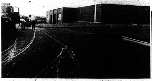
WILL OPEN SOON—Workmen finish an asphalt drive and parking area for the newly constructed Maysville Vocational School which will open for the first time in September. The school, an extension of the State-owned Area Vocational-Technical School at Ashland, will offer courses in five subject areas for a maximum of 150 students. The $300,000 building was financed by Federal and local funds.
