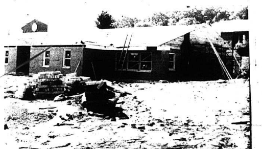
NEW RECTORY-- The above photo shows the rectory which will house the pastor and any volunteers helping with church work at the new Catholic Church under construction in Mt. Vernon.
