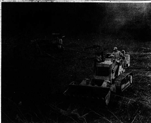
CLEARING THE WAY-- Workers for Bryant and Wilmot of Berea are shown clearing the site of Lake Linville at Renfro Valley. Bryant and Wilmot were the successful bidders for the project at $18,132,000. Clearing is expected to be completed within the near future.
