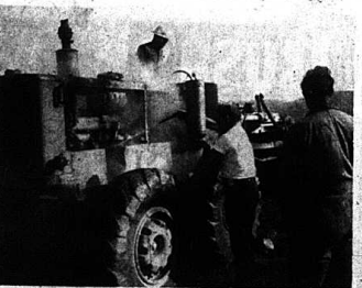
FIRE CHIEF ADDS-- Mt. Vernon Fire Chief John Cox uses a soda and acid fire extinguisher to put out a road grader fire Monday near Renfro Valley. The grader, owned by Greer and young Construction Company of London, caught fire when a crew was doing welding work on it. The city fire department was also called to extinguish a car Saturday afternoon which had caught on fire on Town Hill. The car, which belonged to Dale McClure of Sand Springs was damaged extensively. Later the fire department was called to the home of Londa Lassa off U.S. 150 in Mt. Vernon but upon arriving on the scene found that the blaze consisted of soot burning in the fire. It was unnecessary for the fire department to extinguish the blaze.
