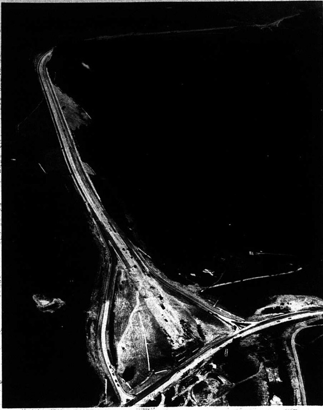
The above aerial photo shows the Interstate 75 bypass around Mt. Vernon, or the "bottleneck" as we have come to be known.
