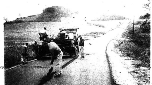
BLACKTOPPING —A three mile stretch of the Scaffold Cane road is presently being blacktopped. The work is almost finished and when completed the road will be blacktopped from Roundstone to the Madison County line. Cantrell Construction Company of Lexington is the contractor.
