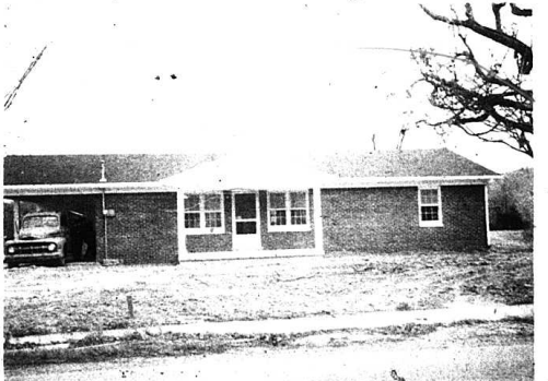
DEDICATED —The new Brodhead Baptist parsonage was dedicated at ceremonies held Sunday afternoon in the basement of the parsonage. The home was erected on the site of the old parsonage which was purchased by Mrs. Ollie Harrison and removed from the site. Rev. John Zupancic is pastor of the church.
