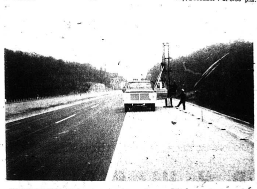
SETTING POSTS —Construction crews drive steel posts in the ground for the guard rails on Interstate 75 by-pass around Mt. Vernon. A hold-up in receiving guard rails has delayed opening the by-pass.
