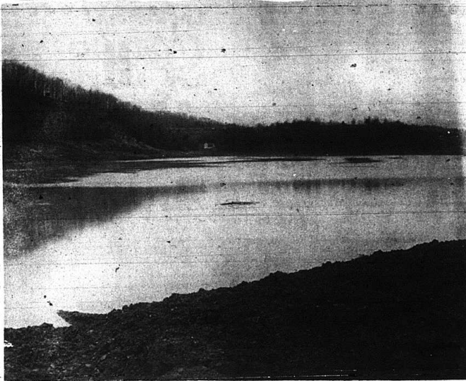
LAKE LINVILLE--Heavy rains Monday night caused this scene at Renfro Valley Tuesday morning. The picture was taken from the partially constructed Interstate-75 Dam at Renfro Valley.
