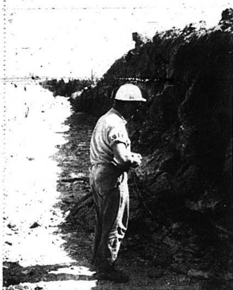
MAKING AN AIRPORT —A construction worker prepares a dynamite blast in the drainage ditch of the runway extension to the Capitol City Airport. The two-phase project includes grading, drainage, and pre-construction for 1968 and final paving for next year. Estimated cost is $1,100,000.
