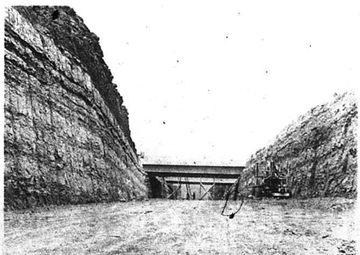
Renfro Road has been re-routed around one end of the dam. Twin bridges span the road for Interstate-75. The road can be used as an emergency spillway should the occasion ever arise. The roadbed is about 13 feet above the regular spillway.
