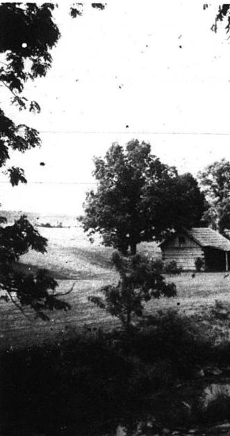
THE BLACKSMITH SHOP at Lincoln Homestead State Shrine near Springfield, Kentucky, is a reproduction of the building in which Thomas Lincoln, father of the 16th President, learned his woodworking trade. It is one of three buildings which the State maintains, on land that was part of the original Lincoln farm. In the Berry House, Nancy Hanks lived during her courtship with Thomas Lincoln. The Lincoln Cabin is a replica of the log house in which the President's grandmother reared her children. Lincoln Homestead State Shrine is five miles north of Springfield on Ky-528.
